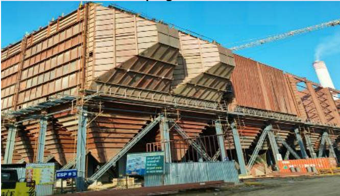
Unit #3 Electrostatic Precipitator Hopper erection work progress
