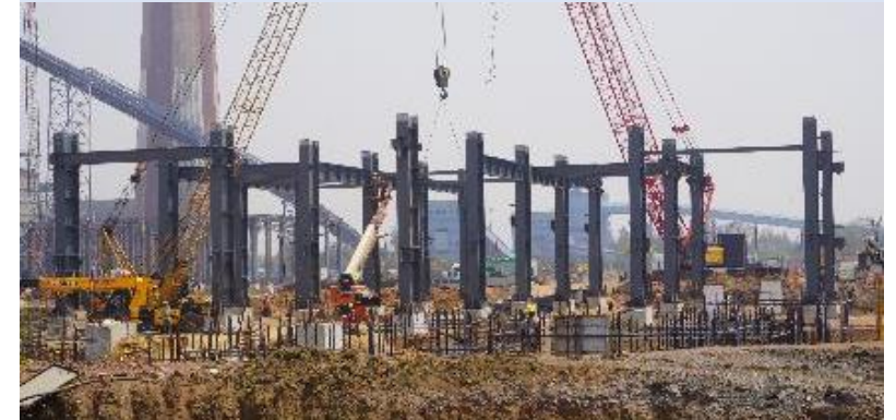
Main Power House and Central Control Room Structure
