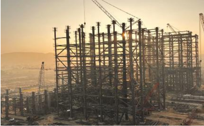
Unit #3 Electrostatic Precipitator Hopper erection work progress
