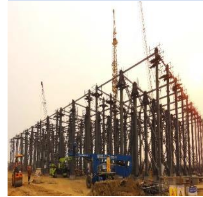
Unit #3 - Electrostatic Precipitator
