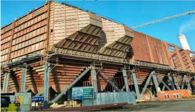
Unit #3 Electrostatic Precipitator Hopper erection work progress
