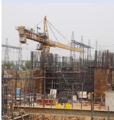
Unit #3 - Turbine Generator Deck
