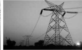
Longest Private HVDC Line in Asia
