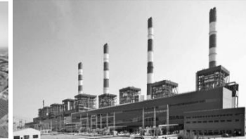
Largest Single Location Private Thermal IPP
