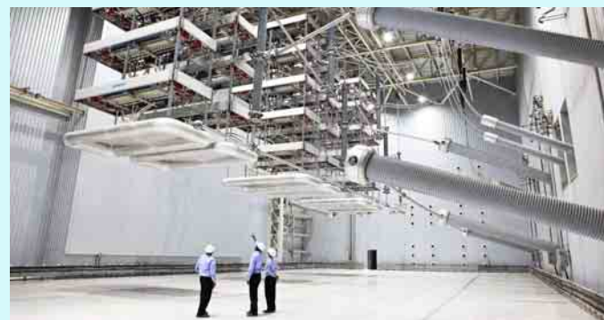
One of the power plants at the giant Mundra port development, where Chinese firms have been key suppliers. Photo: SCMP Pictures
