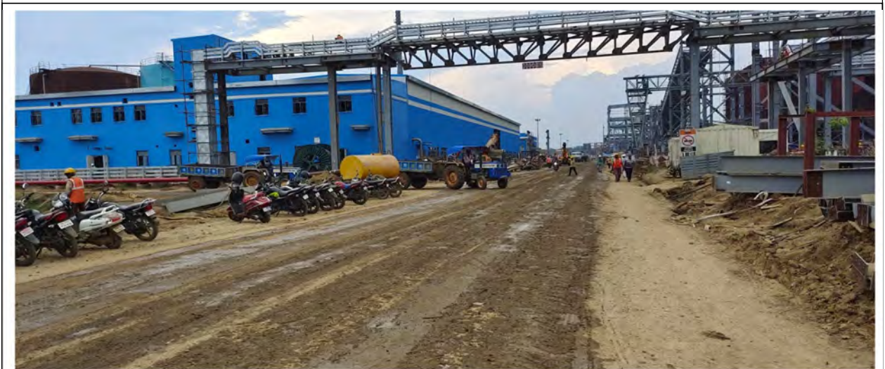
Water sprinkling on road to reduce fugitive emission
