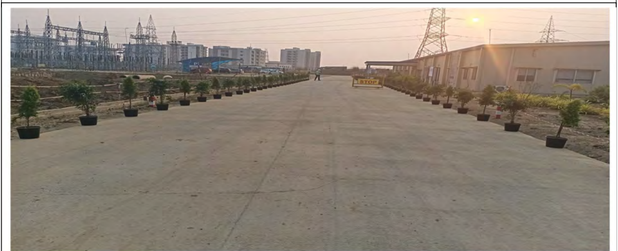
Concrete Road which help to reduce fugitive emission
