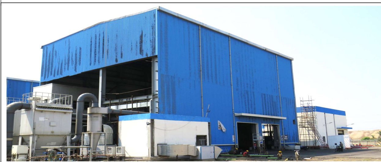
WAGON TIPLER WITH DUST EXTRACTION SYSTEM
