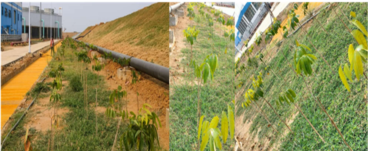
Green Belt Development along the Ash Dyke
