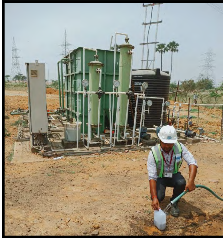
Figure 11: Water Sampling at STP Outlet plant
