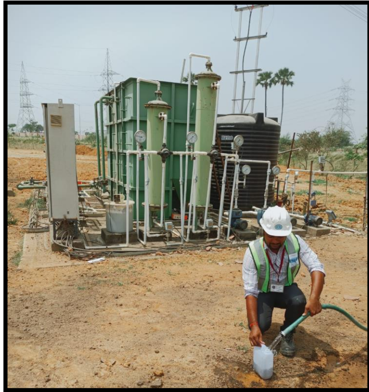
Figure 11: Water Sampling at STP Outlet plant
