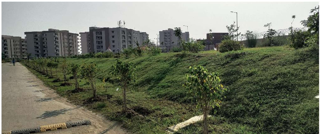
Green Belt Development in Progress
