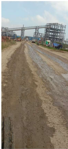
Water sprinkling on road to reduce fugitive emission
