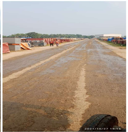
Water sprinkling on road to reduce fugitive emission
