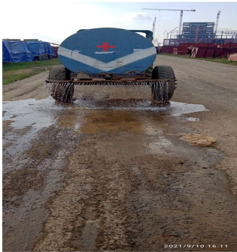
Water sprinkling on road to reduce fugitive emission
