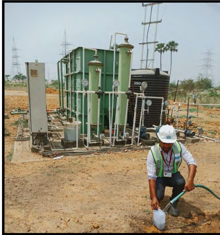
Figure 11: Water Sampling at STP Outlet plant
