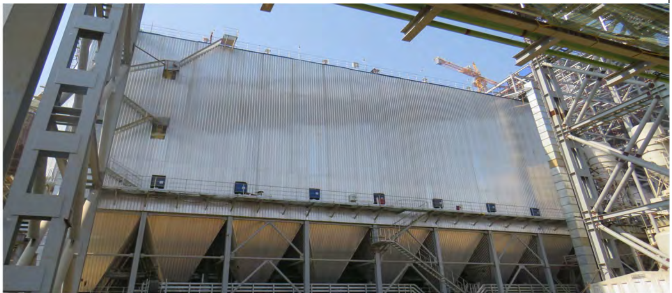
Electro Static Precipitator (ESP)
