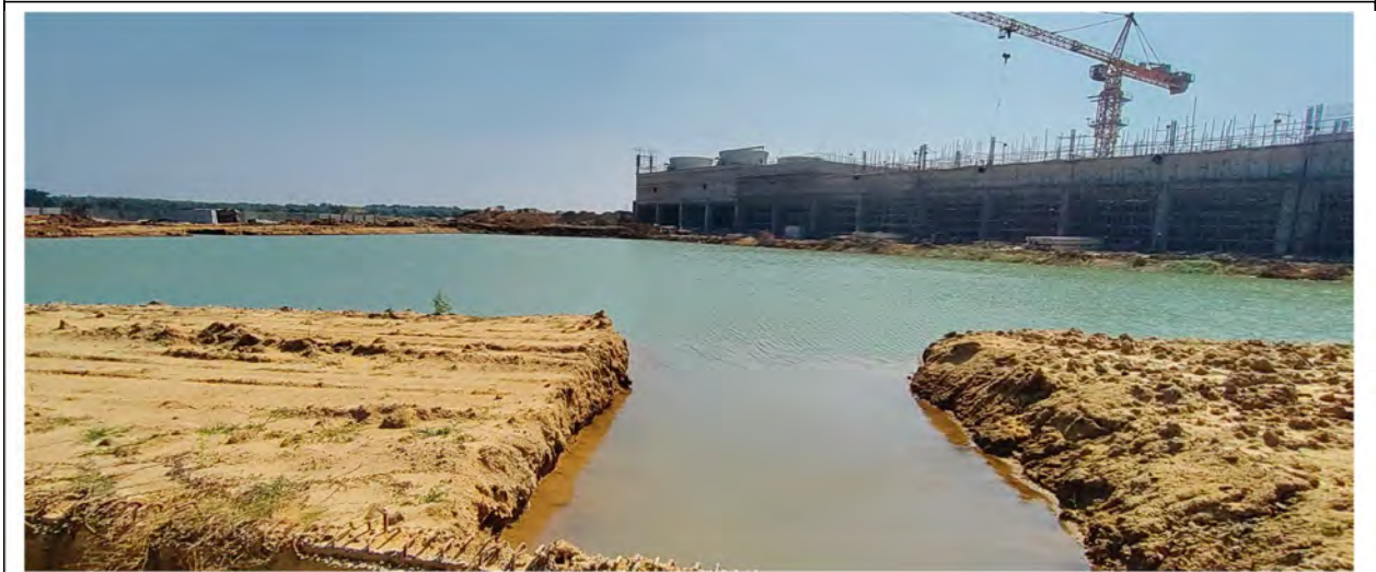
Rain Water Harvesting Pond
