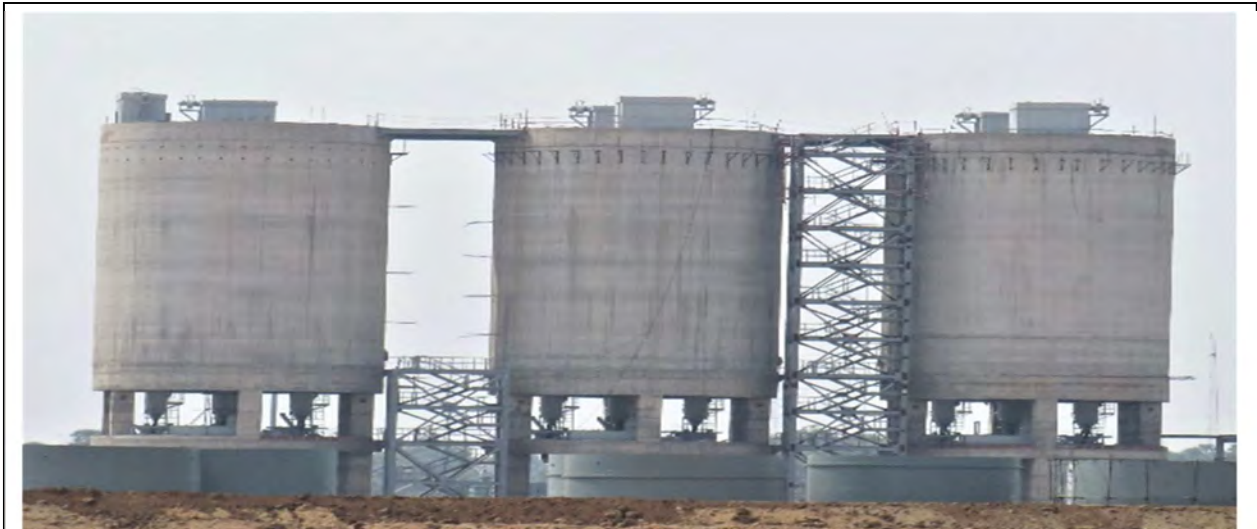
Fly Ash Silo with Bag Filter
