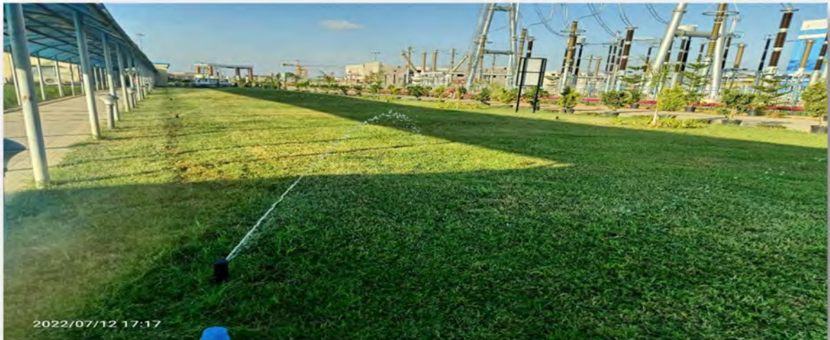
Green Belt (inside plant)
