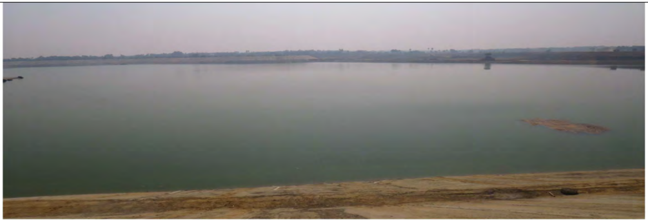
Raw Water Reservoir
