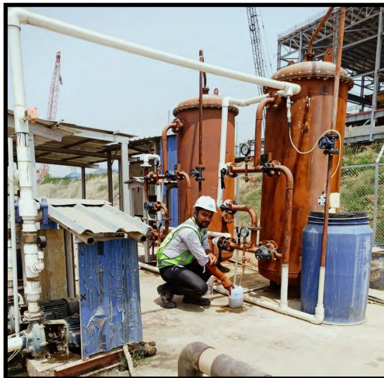
Figure 12: Water Sampling at STP Outlet township
