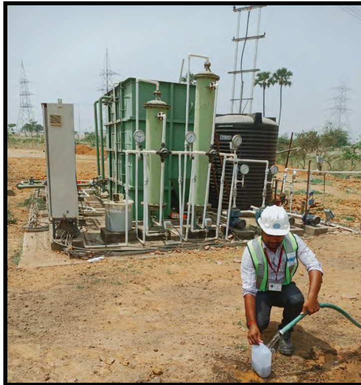
Figure 11: Water Sampling at STP Outlet plant
