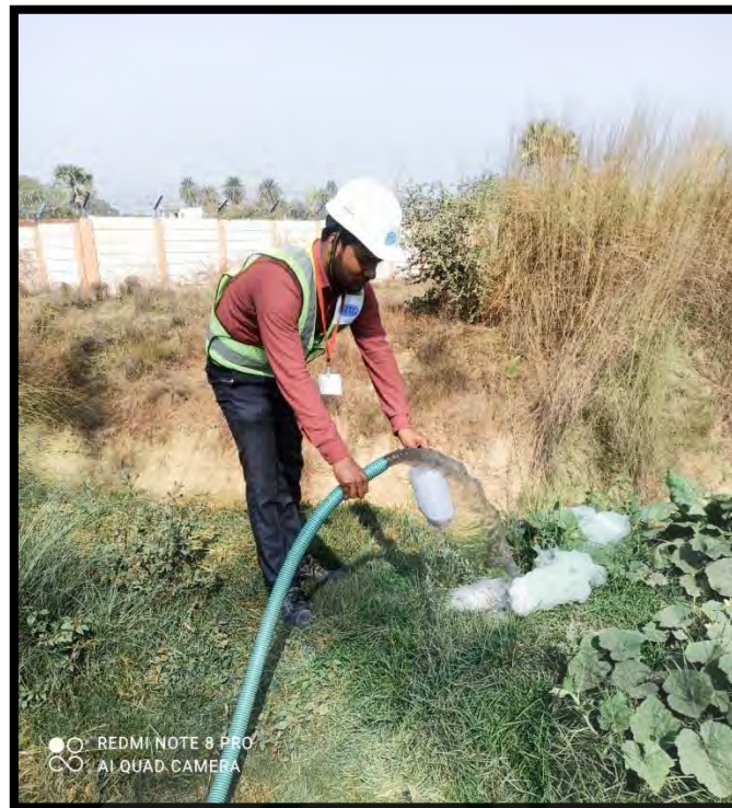
Figure 11: Water Sampling at STP Outlet plant
