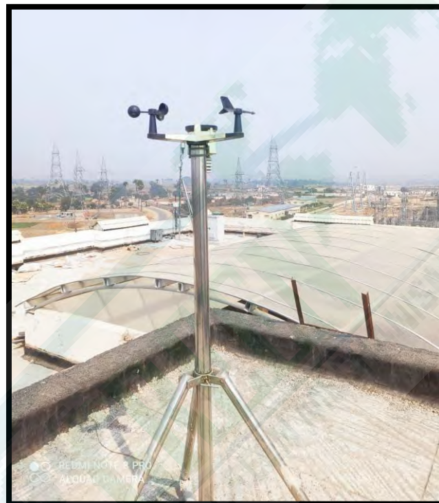
Figure 1: Weather Monitoring Station at Hostel Block
