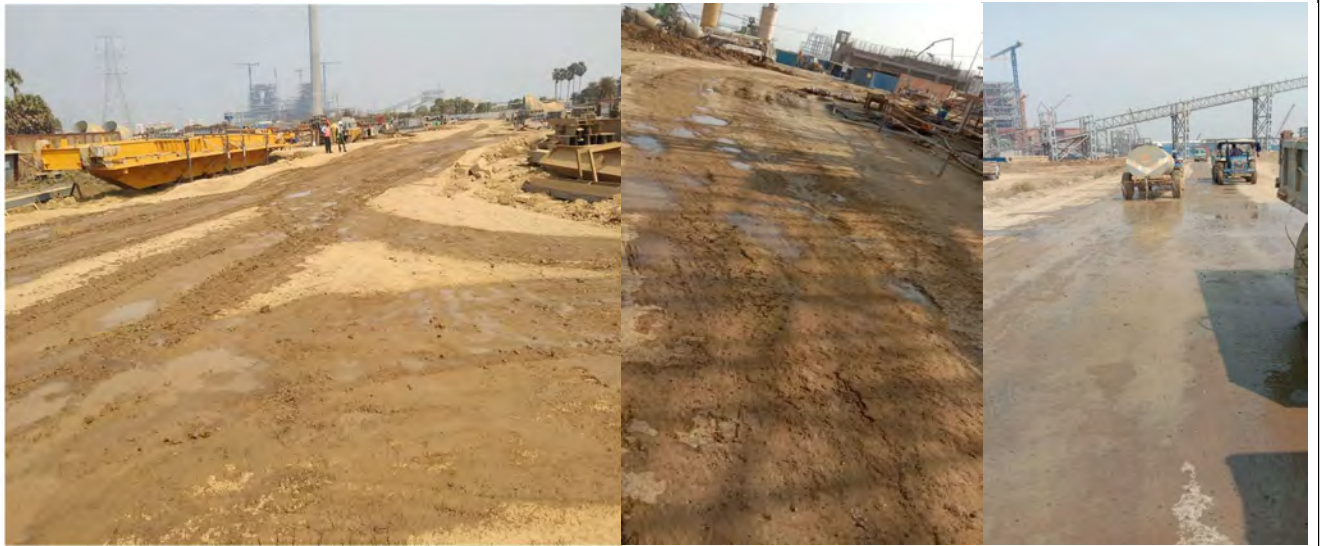
Water sprinkling on road to reduce fugitive emission
