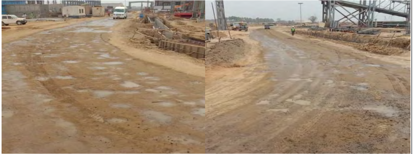
Water sprinkling on road to reduce fugitive emission
