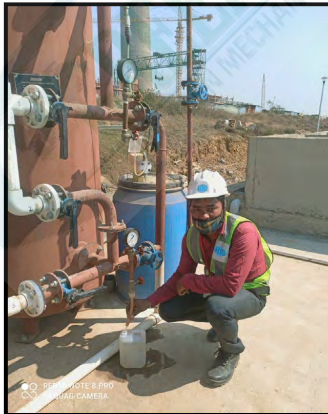
Figure 12: Water Sampling at STP Outlet township
