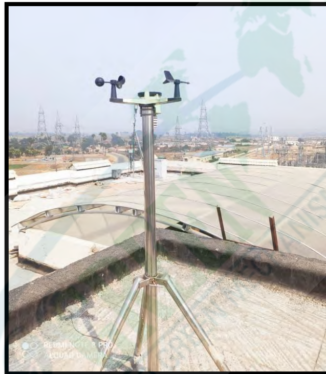
Figure 1: Weather Monitoring Station at Hostel Block
