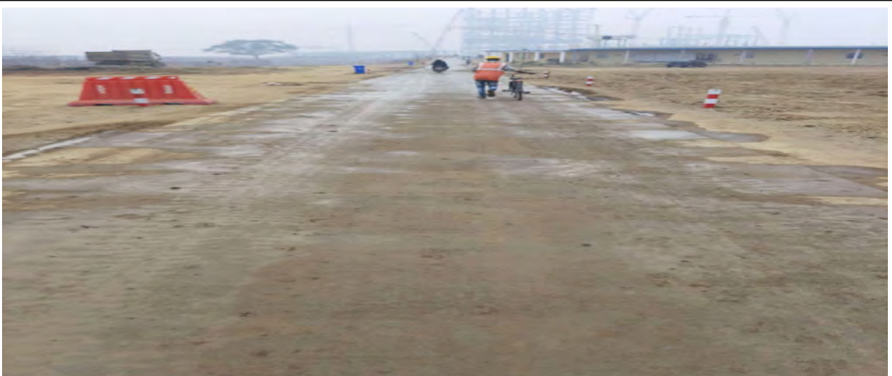
Wet internal road after water sprinkling
