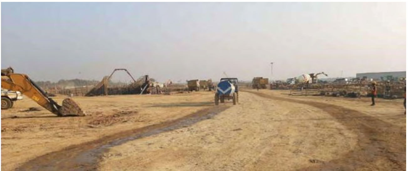
Water Sprinkling at Site
