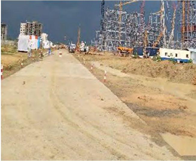
Construction of RCC Roads to easy movement and reduce fugitive dust emission
