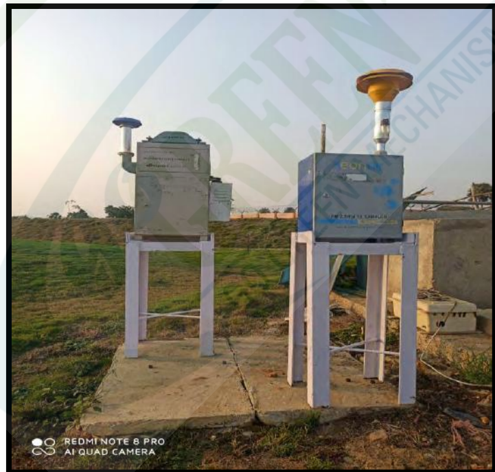
Figure 6: Ambient air Monitoring Near Motia Village
