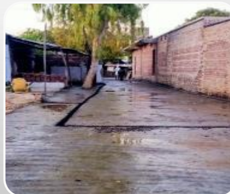
CC road construction @Aton
