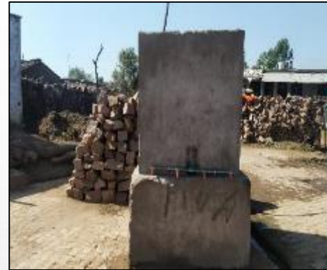
Water tank for irrigation
