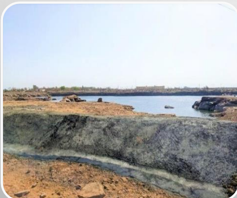
Pond Deepening -Embankment
