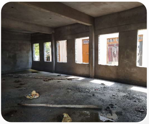
Library construction @Aton
