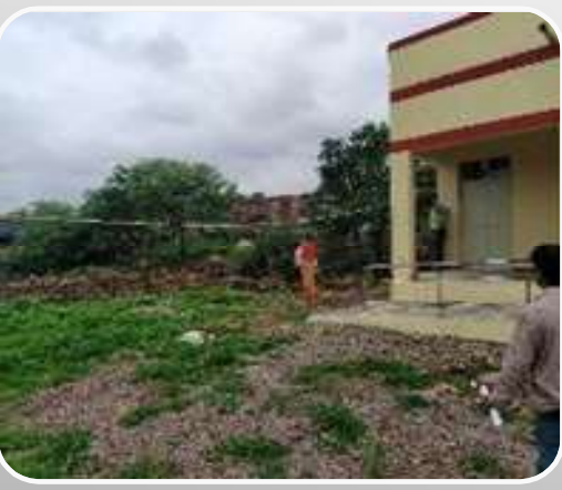
Classroom construction site @ Haniheda
