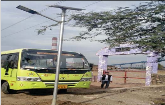
Street light in vicinity villages
