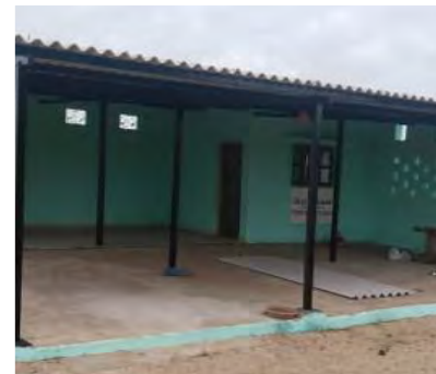
Renovation of Shed at Shekranpir Bhopavandh - 2000+ Benefited
