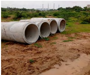
4 location Pipe Support – 4800+ Benefited
