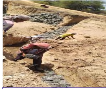
Construction of Pipe Culvert – 400+ Benefited
