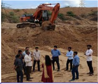
Restrengthening & Desilting of Check dam – 720+ Benefited
