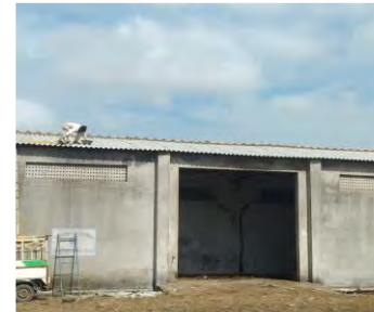
3 Villages - Renovation of Godown and Gashala Shed
