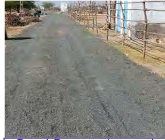
Road Renovation and Civil Maintenance Work at Fisherman Vasahat – 600+ Benefited
