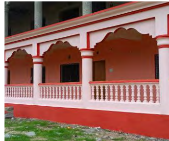
Renovation of High School at Zaarapa – 2200+ Benefited
