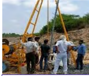
6 Percolation Bore well Recharge – 4000+ Benefited
