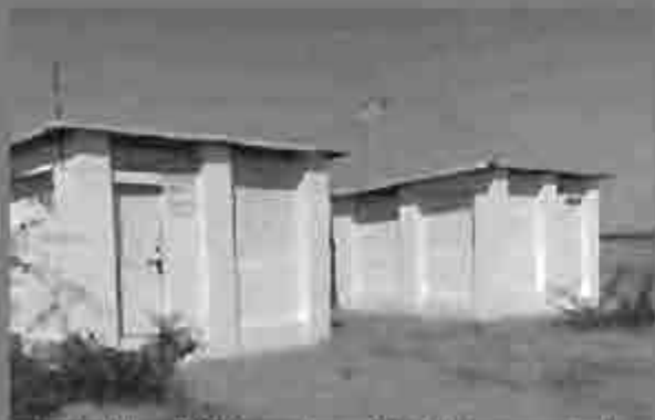
Painting & Branding Old Structure at Old Bandar and Luni Bandar
