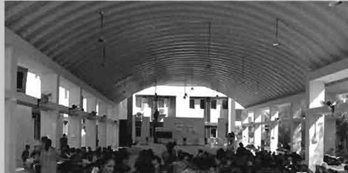
Construction of Prayer Shed at AVMB
