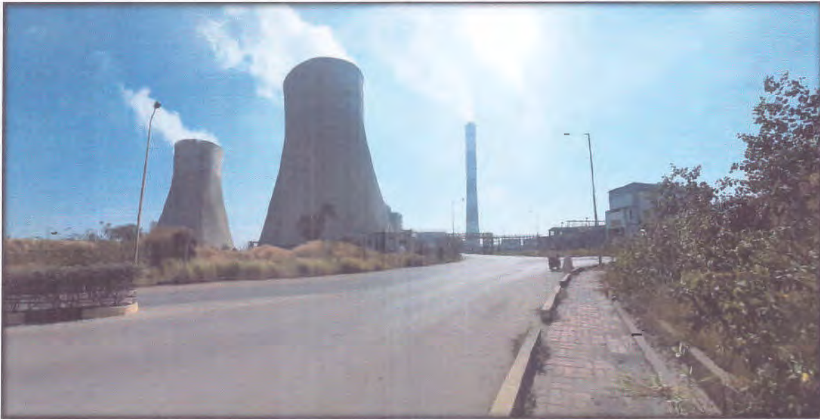
Figure No.1.Raipur Energen Limited.
