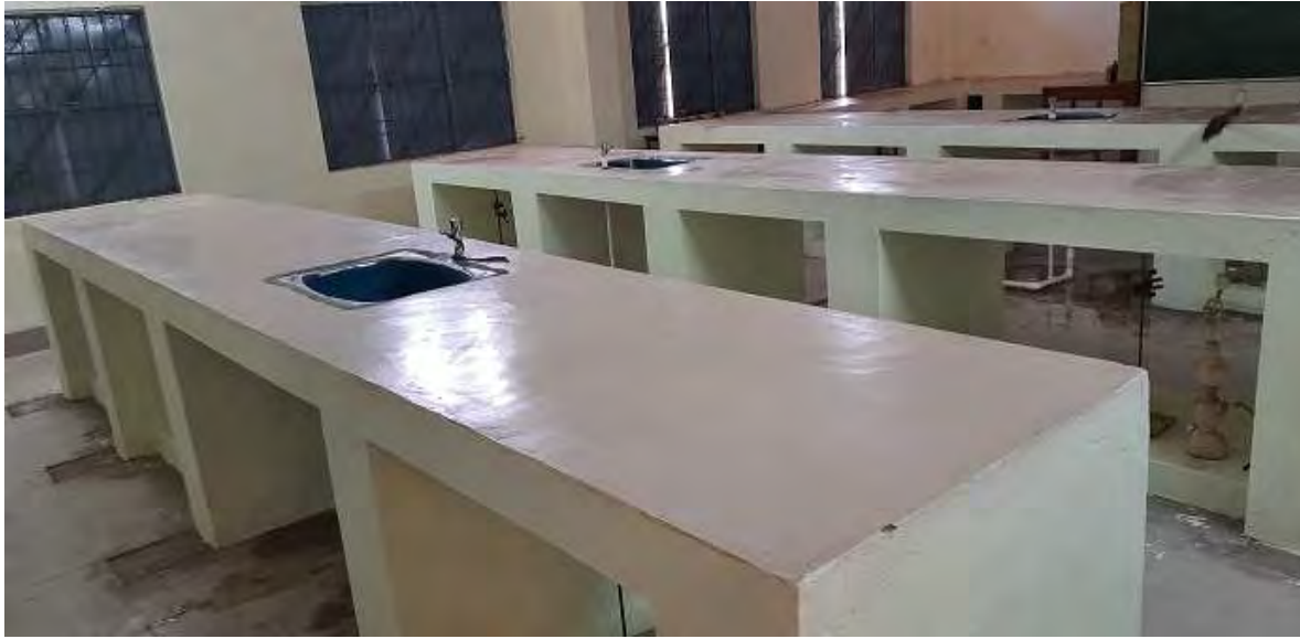
Construction of Science Lab. platform at PG College
