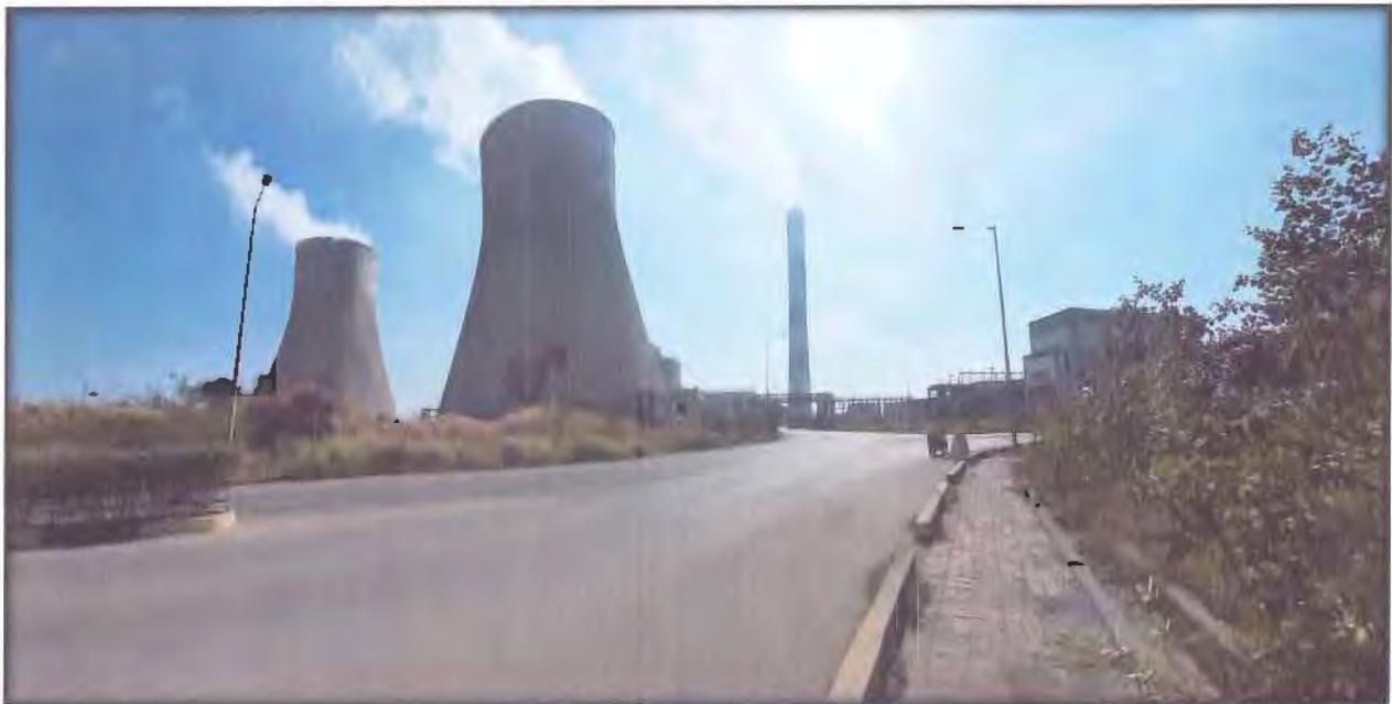
Figure No.1. Raipur Energen Limited.
