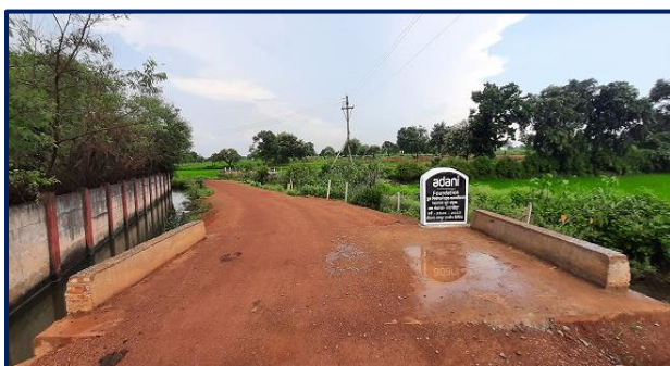
Murra Bhatapara Road Repair & Culvert Construction
