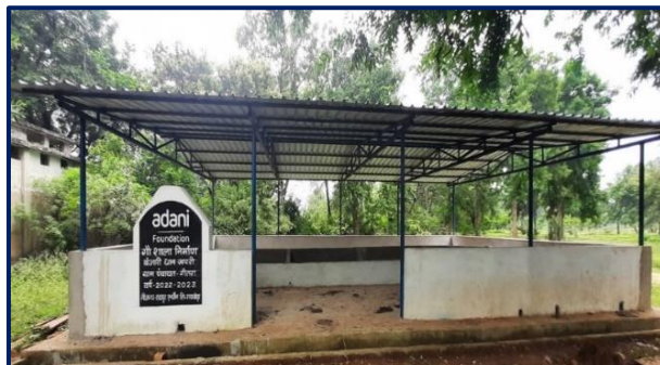
Gaushala Shed -Banjari -Khapri
