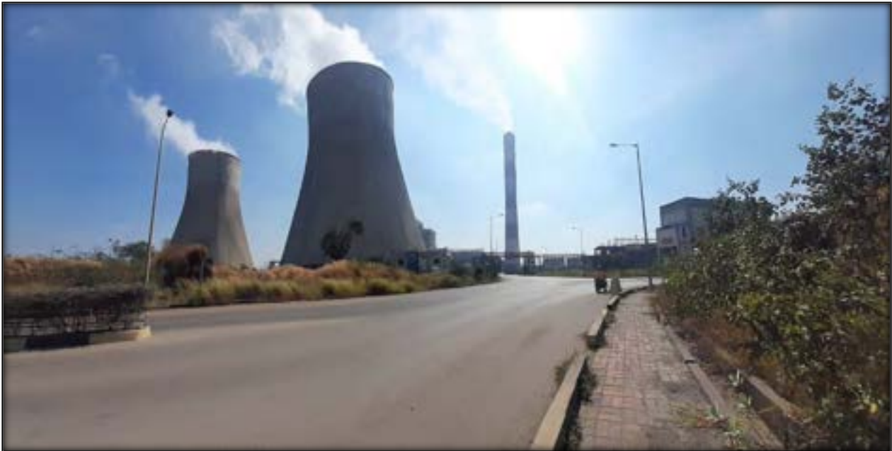
Figure No.1 M/s Raipur Energen Limited
