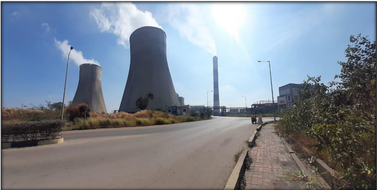
Figure No.1. M/s Raipur Energen Limited
