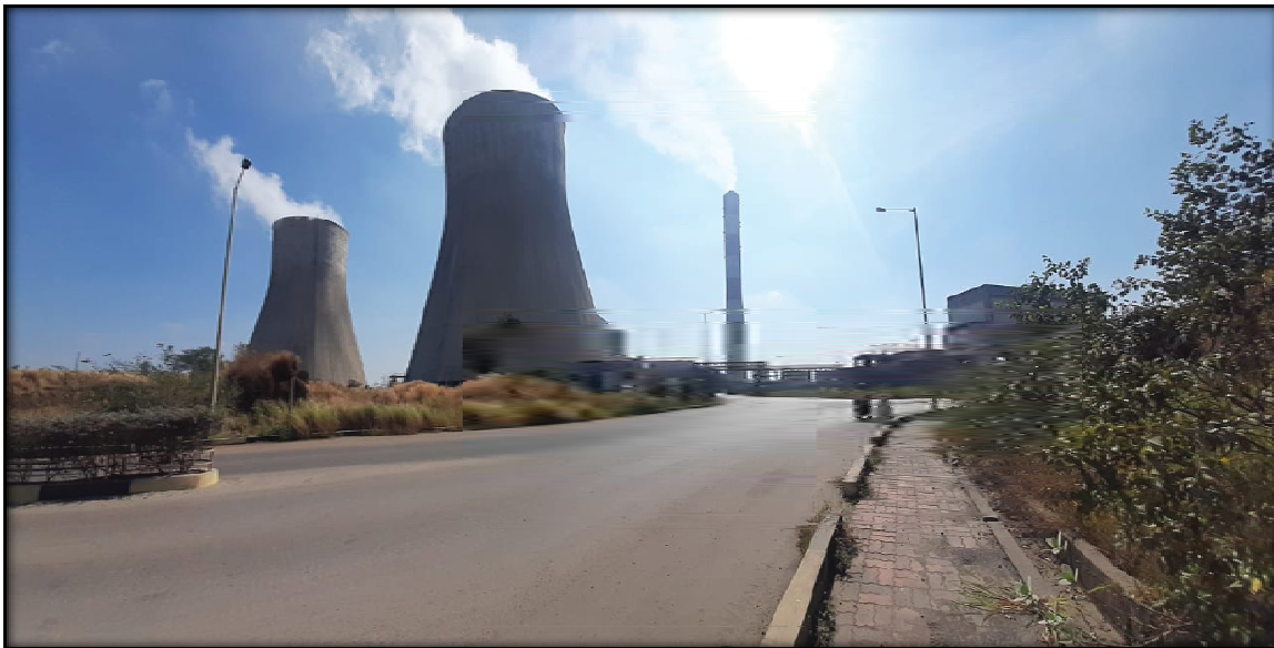
Figure No.1. Raipur Energen Limited.
