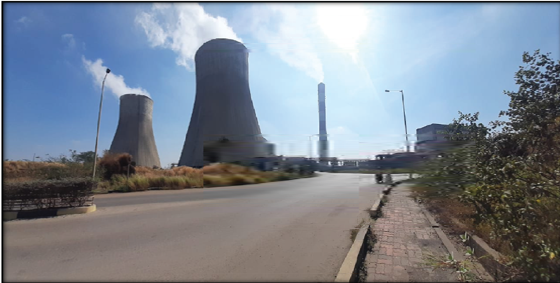
Figure No.1. Raipur Energen Limited.
