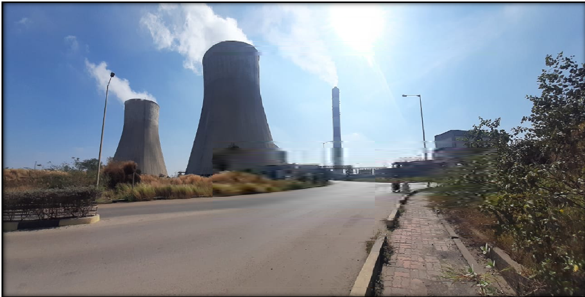
Figure No.1. Raipur Energen Limited.
