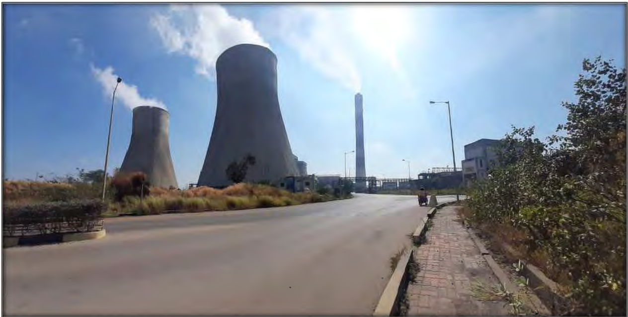
Figure No.1. Raipur Energen Limited.
