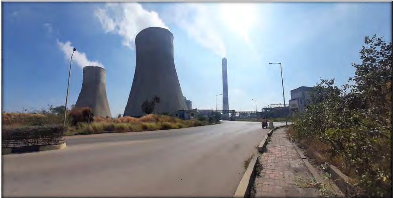
Figure No.1. Raipur Energen Limited.
