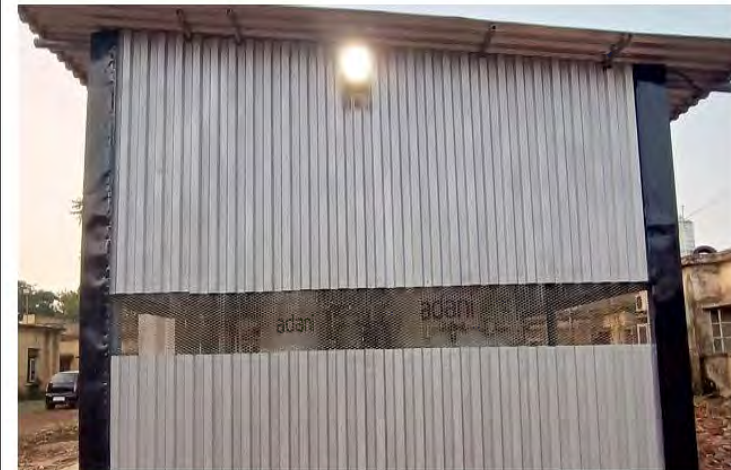
Oxygen Plant Shed – CHC Tilda
