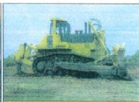
Soil and OB removal by Ripper Dozer
