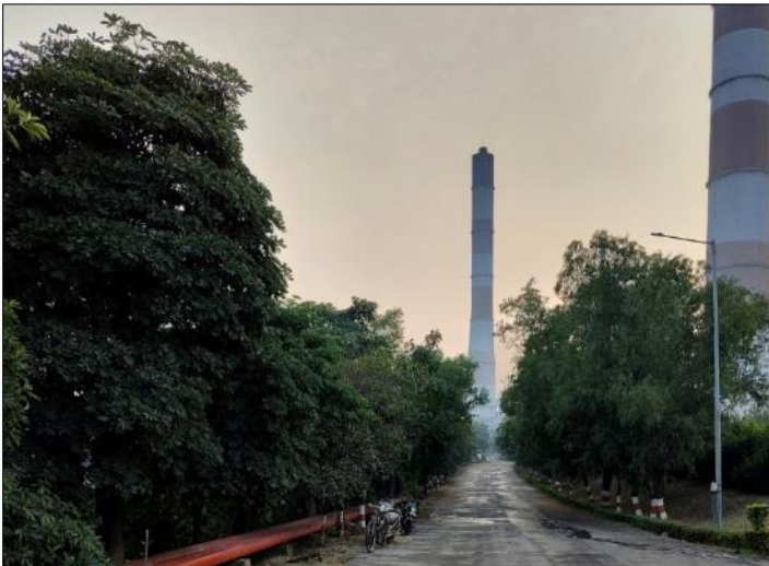
DM Plant Road
