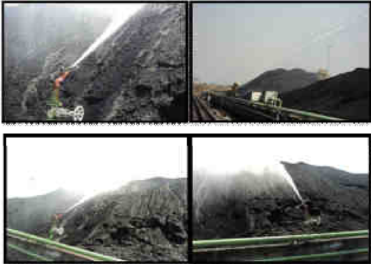
Fig. 10: Rain Guns at Coal Yard for Reduce Fugitive Dust Suppression
