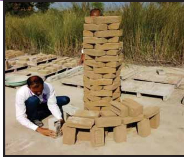
Dry Bricks Ready for Furnace
