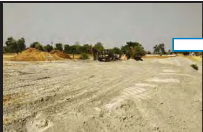
Ash Compaction & Chaining
