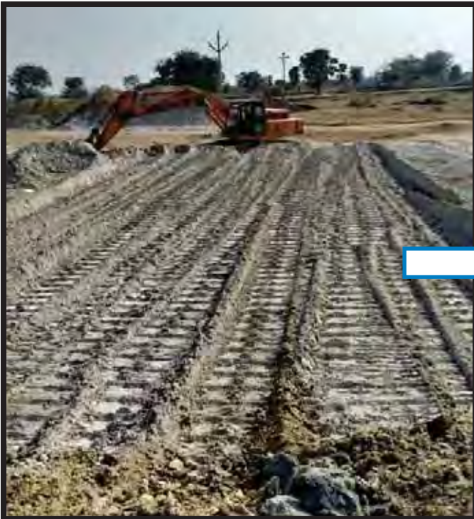
Ash Compaction & Chaining
