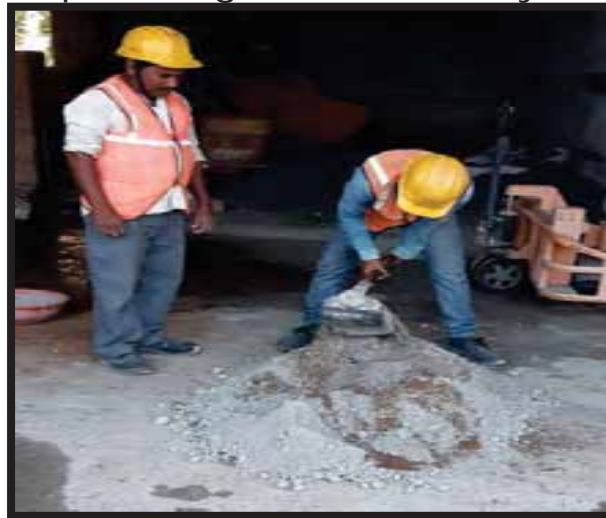
Mixing of Bottom Ash with Clay
