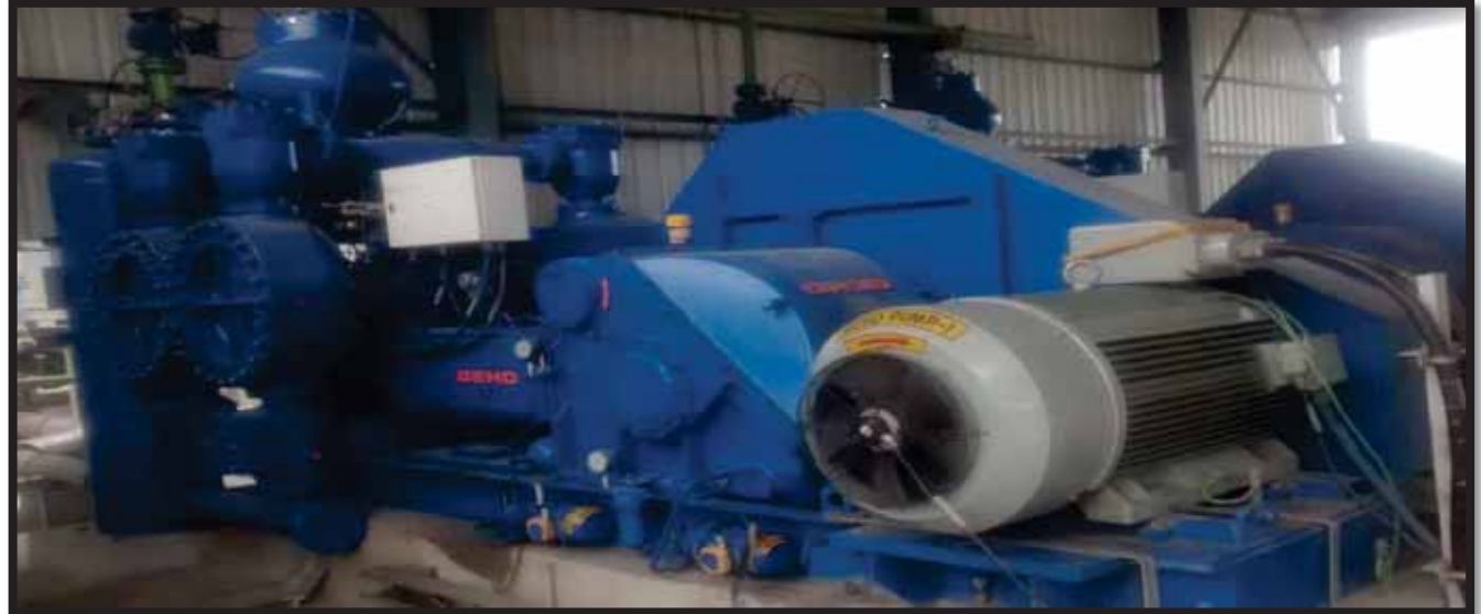
HCSD pump (GEHO) (Cap-237 M 3 /hr, 40 bar) - Qty 2 no's.
