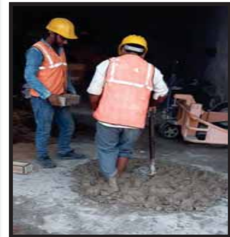
Moulding of Fly/ Bottom Ash with Soil
