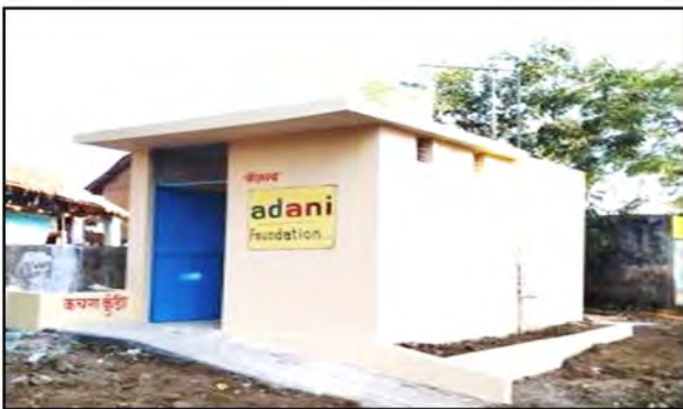
Berdipar School Toilet
