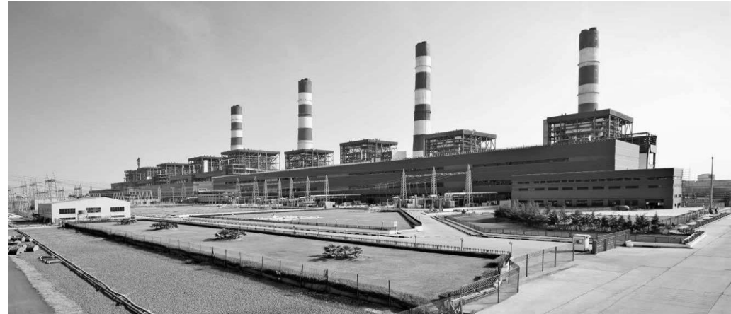
External view of the plant
