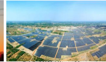
648 MW Ultra Mega Solar Power Plant
