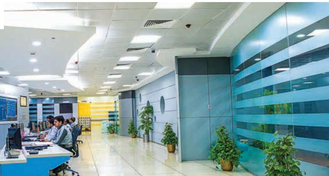
Our Power Plant Control Room.
