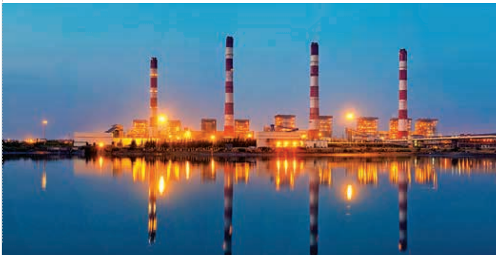
Night view of 4,620MW Mundra plant.
