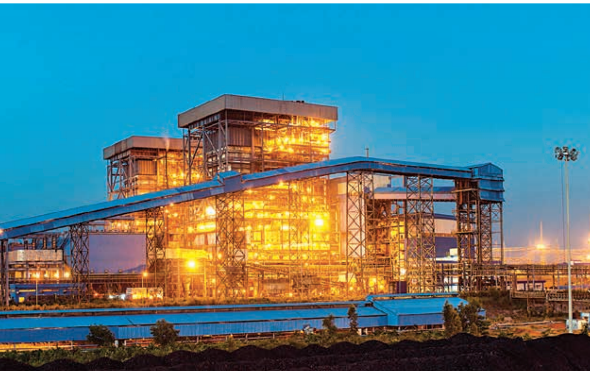
1,200MW UPCL power plant at Udupi, Karnataka.
